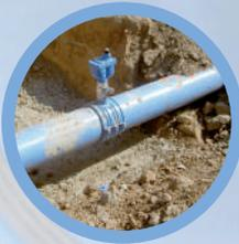
**Tapping saddles** allow connecting the pipe in the perpendicular direction to all kinds of fittings, being available with screw ends and flange ends
