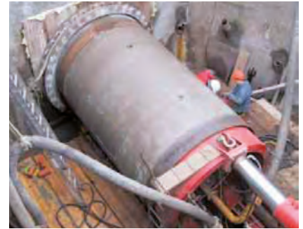
Polymer concrete (pipe jacking).
