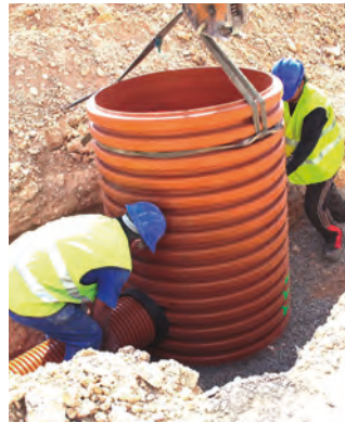
PIPING INSTALLATION TO THE MANHOLE BODY.
