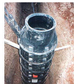
INSPECTION MANHOLES USING PLASTIC MATERIALS (POLYESTER AND POLYETHYLENE)
