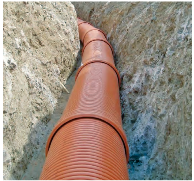
SANECOR® 1200 MM PIPING WITH ANGULAR DIVERSION.
