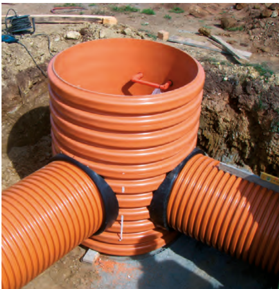
MANHOLE INSTALLATION IN COLLECTORS WITH DIRECTION CHANGE.
