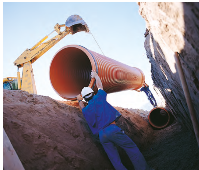
SANECOR® PIPING INSTALLATION IN GALLERY AND TRENCH.
