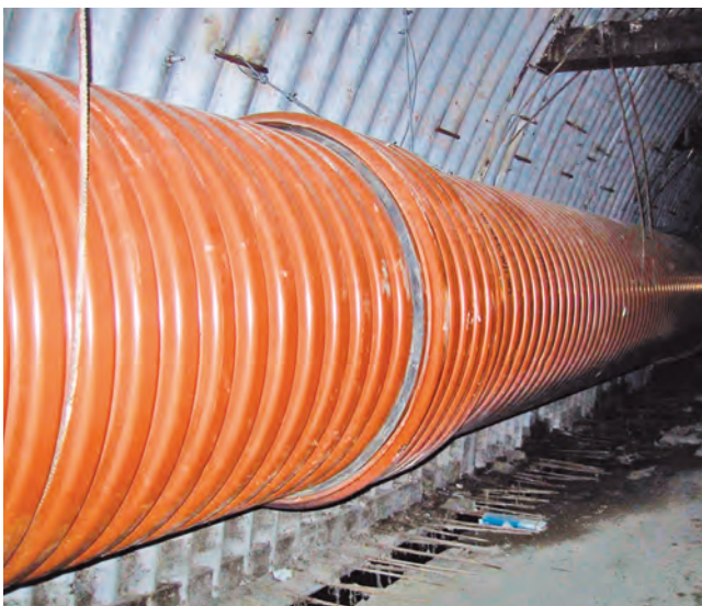
SANECOR® PIPING INSTALLATION IN GALLERY AND TRENCH.
