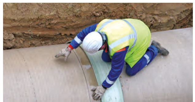
LARGE-DIAMETER PRFV PIPING SLEEVE JOINTS.
