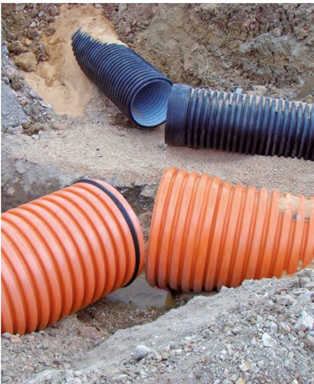
CORRUGATED PVC PIPING (ORANGE) AND CORRUGATED PE (BLACK).
