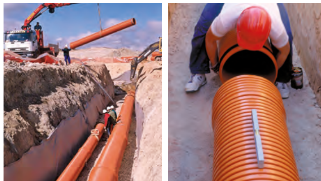
LEFT, SANECOR® PIPING INSTALLATION WITH DISCRETE MECHANICAL MEANS (MEDIUM AND LARGE DIAMETERS), RIGHT, MANUAL CONNECTION (SMALL DIAMETERS).
