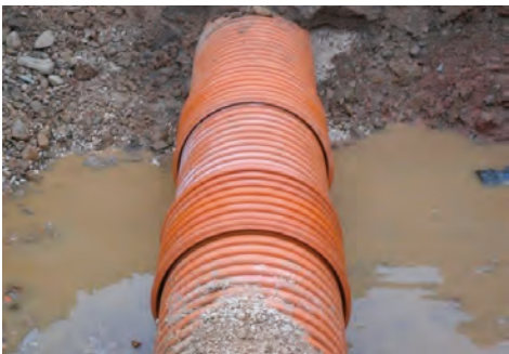
SANECOR® HAS A VERY WIDE RANGE OF SPECIAL FITTINGS UP TO DN1200 (LEFT, REPAIRS WITH SINGLE SOCKET).
