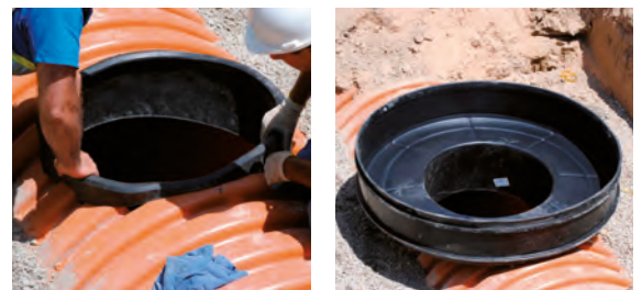
MANHOLE BODY INSTALLATION WITH INSPECTION BASE.
