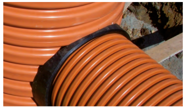
SEALED CONNECTION IN SANECOR® MANHOLES.
