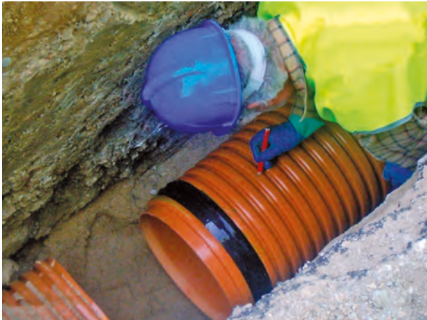
MANUAL CONNECTION OF CORRUGATE PIPING.
