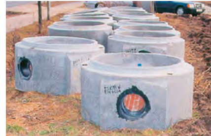
INSPECTION MANHOLES IN CONVENTIONAL MATERIALS (CONCRETE AND BRICK), ON THE RIGHT, PREFABRICATED CONCRETE RINGS.
