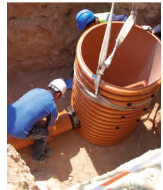
PIPING INSTALLATION TO THE MANHOLE BODY.
