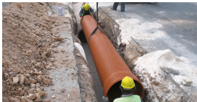
ONSITE HANDLING OF SANECOR® PIPING.
