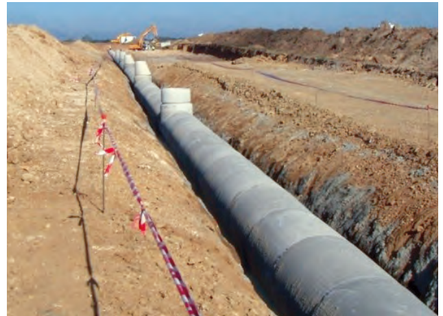
REINFORCED CONCRETE COLLECTOR.
