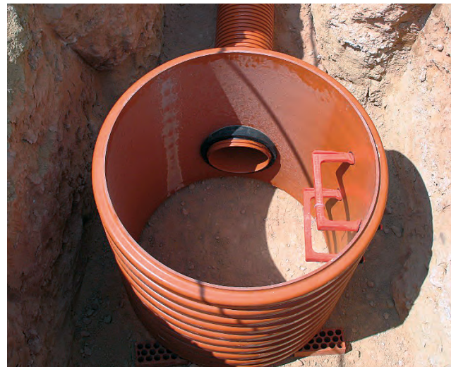
MANHOLE BOTTOM CONCRETING, FIRST PHASE.
