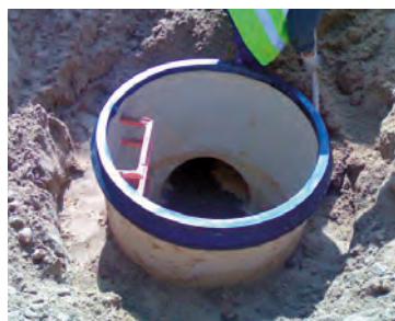
INSPECTION MANHOLES USING PLASTIC MATERIALS (POLYESTER AND POLYETHYLENE)
