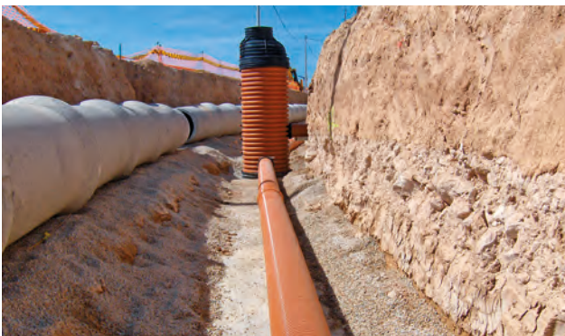
SANECOR® CONCRETE COLLECTOR MANHOLES FOR WASTE WATER WITH A RAINWATER COLLECTOR
