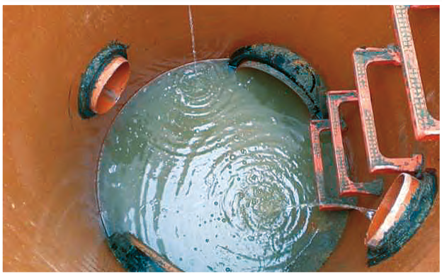
EXECUTING MULTIPLE CONNECTIONS IN SITU.
