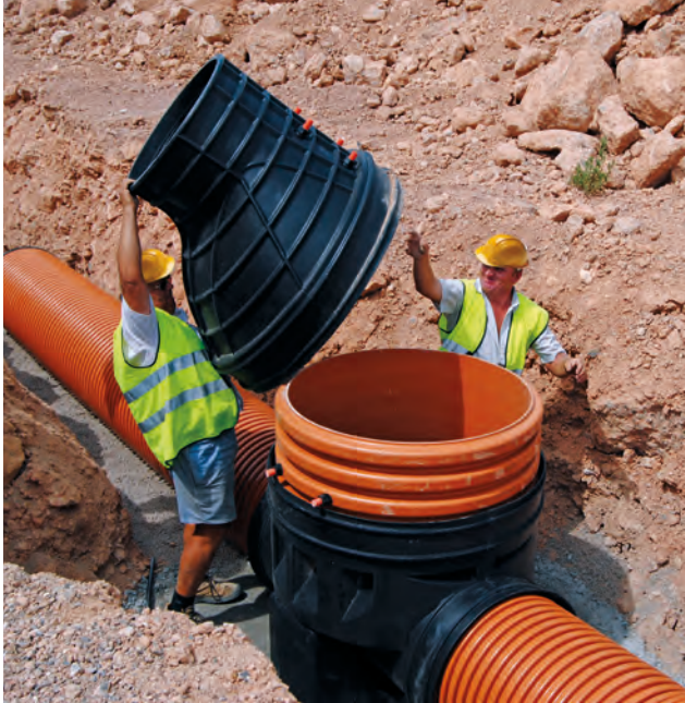
FULL PASS-THROUGH CONNECTION PART INSTALLATION.
