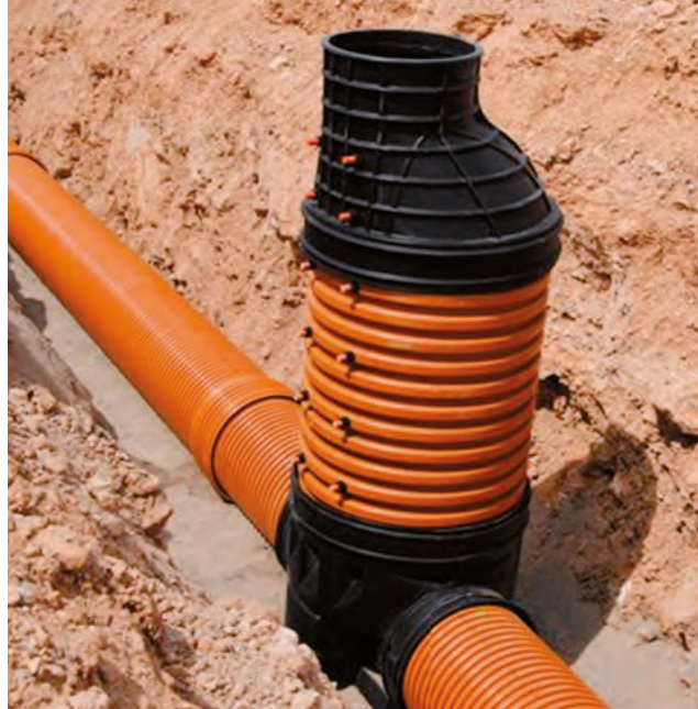
FULL PASS-THROUGH CONNECTION PART INSTALLATION.
