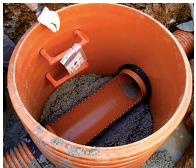
MANHOLE BOTTOM CONCRETING, SECOND PHASE.
