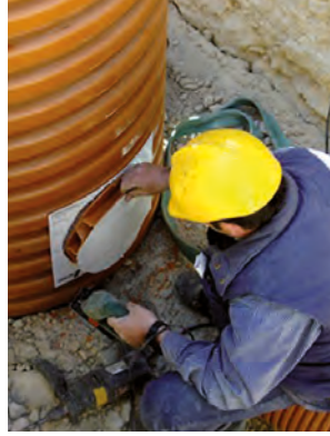
HOLE DRILLING PROCEDURE FOR ELASTOMER CLIP INSERTION.
