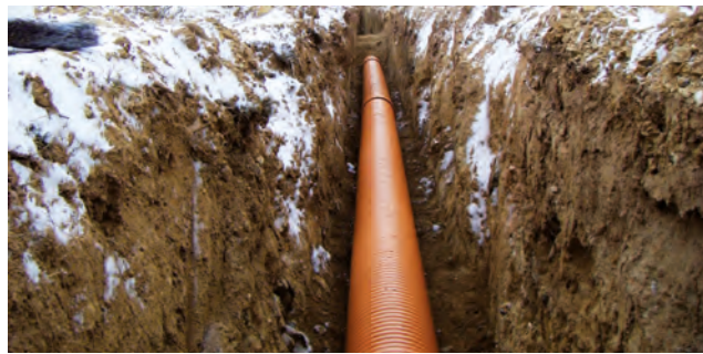
VIEW OF SANECOR® PIPING INSTALLED IN A TRENCH.
