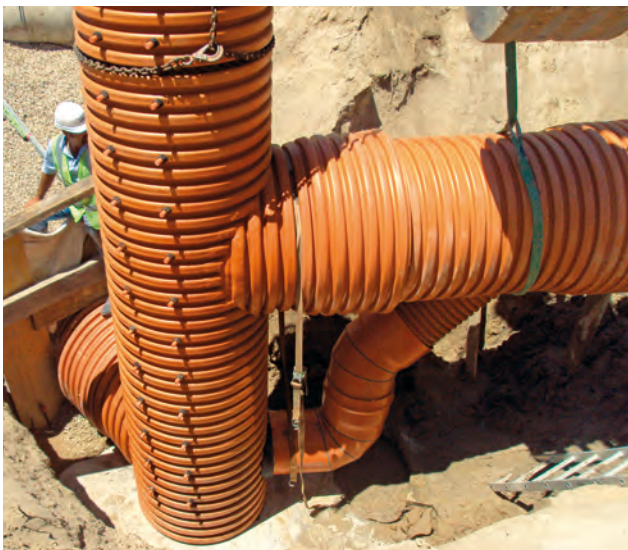
CASCADING MANHOLES WITH THE SANECOR® MANHOLE SYSTEM (MADRID TYPE ON THE LEFT).
